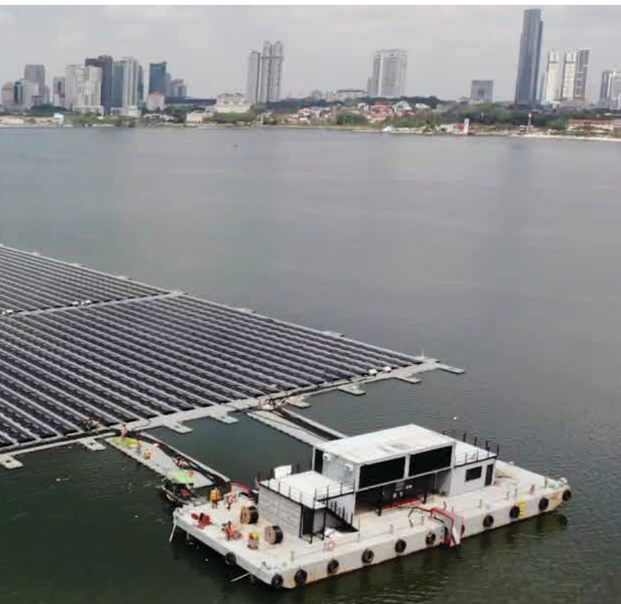
Offshore Floating Solar Farm, Woodlands Senoko
