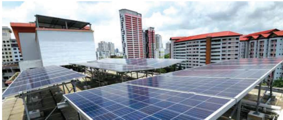
Solar Panel installation at Toh Guan
