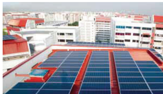
Solar panels on top of a HDB building
